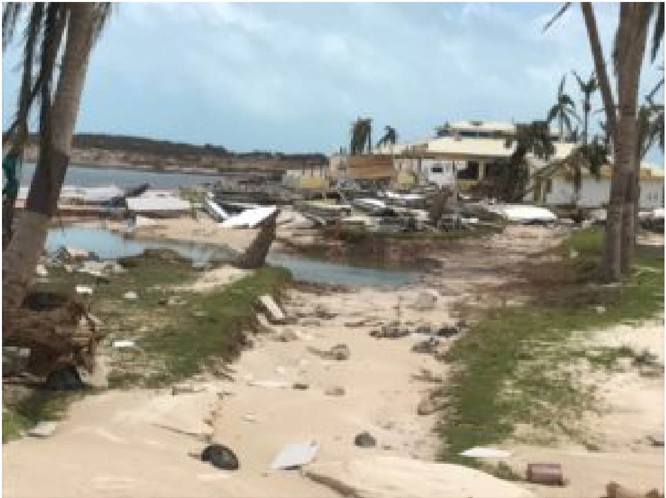
Club Orient Resort – damage to beach, Papagayo restaurant and other buildings
