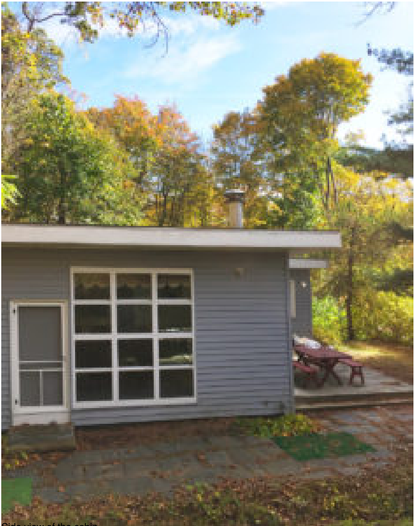
Side view of the cabin
